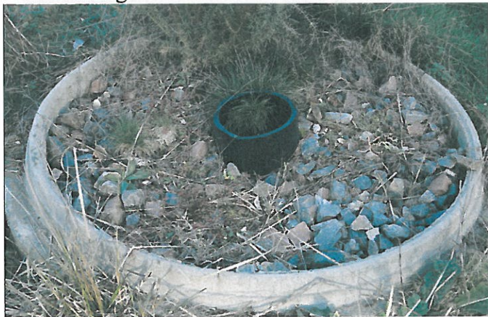
Event de biogaz
